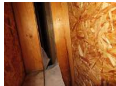
Photo 16: Parapet Wall Composition, (looking down) [Photo by Juxta, 2025]
