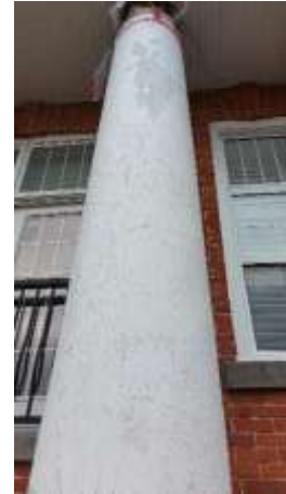
Photo 6: Cracking of Parging and Peeling Paint, Column 3
