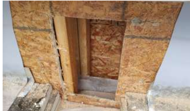
Photo 13: Parapet Wood Framing at Exploratory Opening
