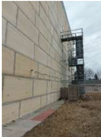
Photo 2: Cement Boards and Scaffold Egress Stair, West Elevation
