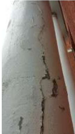
Photo 5: Cracking of Parging, Column 3
