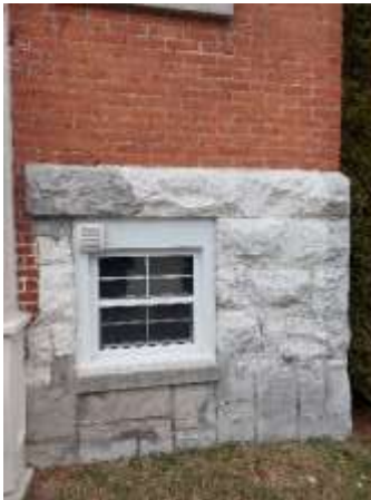
Photo 1: Masonry Cracking and Previous Repairs, Southwest Corner
